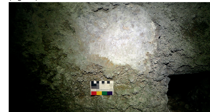
Fig. 5A. A portion of surviving bright white waterproof lining on the wall of the pool of the caldarium .
