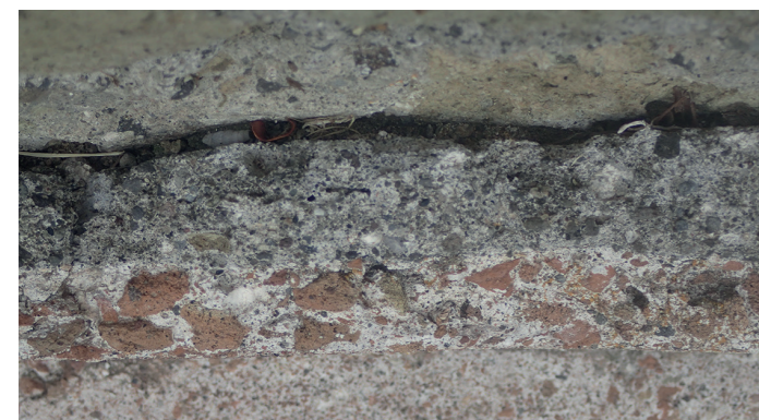
Fig. 1. The two distinct layers of the waterproof linings in Herculaneum: a bottom preparatory layer with volcanic aggregate and top water interfacing layer with crushed terracotta aggregate.
