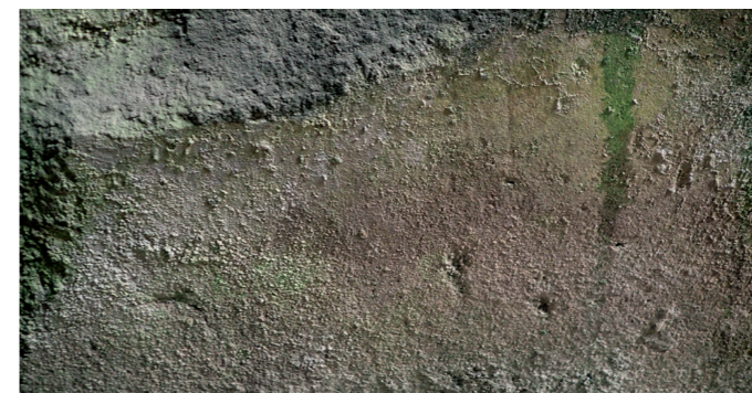
Fig. 4B. The cocciopesto wall lining of the cruciform natatio with finely reduced terracotta aggregate.
